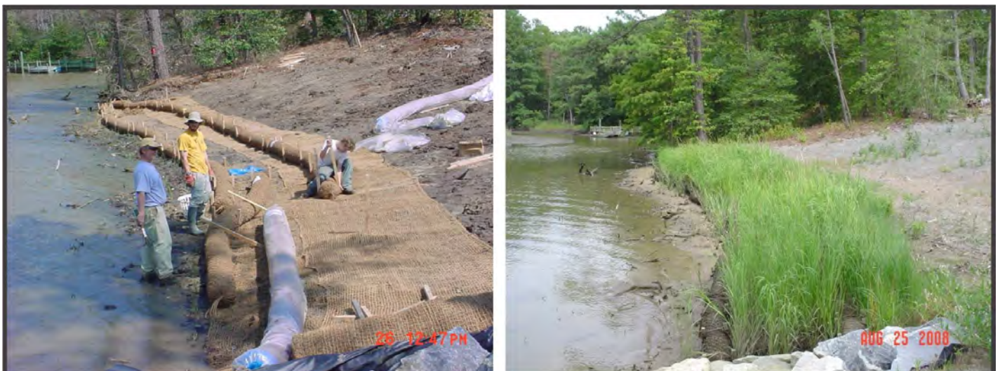
Figure 3-2. Coir logs and mats placed at toe of a graded bank for temporary stabilization while planted tidal marsh and riparian buffer become established. Photos by P. Menichino.
