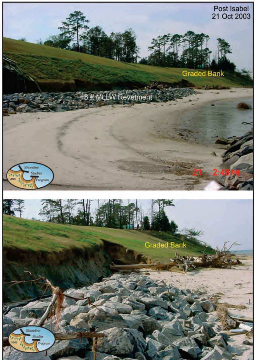
Figure 3-9. Revetment on the James River that was overtopped by storm surge and waves during Hurricane Isabel. Photo dates 21 October 2003.
