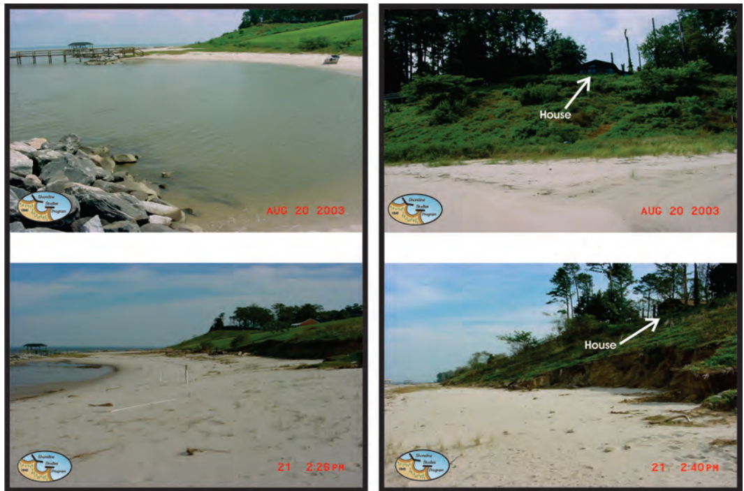
Figure 4-12. Van Dyke ground photos before (top) and after (bottom) Hurricane Isabel (from Hardaway et al., 2005).
