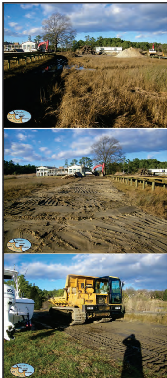
Figure 5-13. Photos taken during construction at Captain Sinclair's Recreational Area on 29 Jan 2016.
