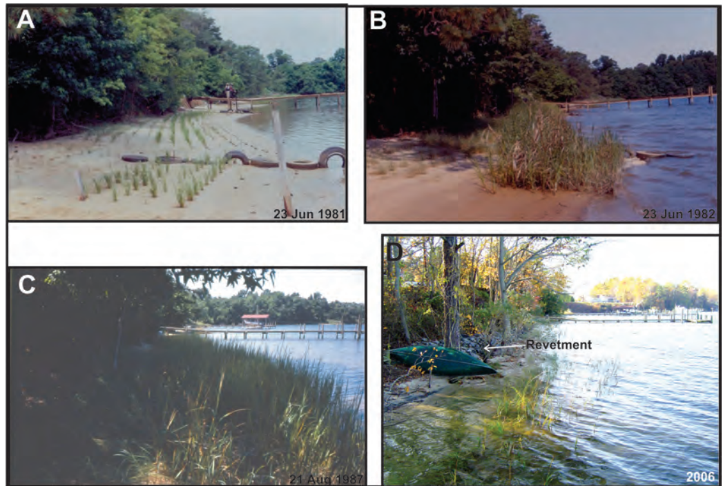
Figure 4-1. Lee marsh management site A) just after installation, B) a year later, C) six years after installation, and D) 25 years after construction.
